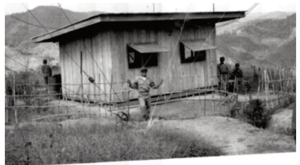
Mountain top communication stations that need regular maintenance visits from EMD technicians.
